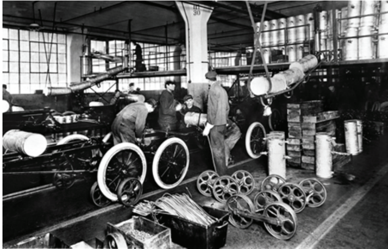
The Highland Park assembly line, 1913. All images courtesy Ford Motor Company.
